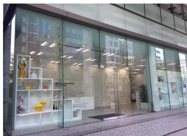
Entrance facing Meiji Street
